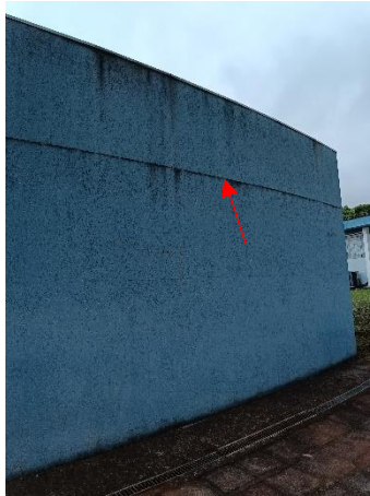
Figura 126: Bolor – Fachada C
